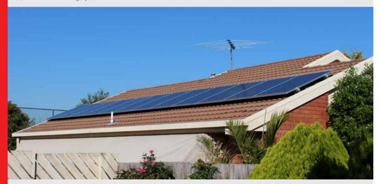
/ This 3kW PV system was installed on a single-family home in a suburb of Melbourne, Australia. The PV system has been designed to cover an average daily consumption of 8-9kWh. During winter and on cloudy days the system provides most of the daily usage. In summer, the output of the system is almost double the self-consumption.
